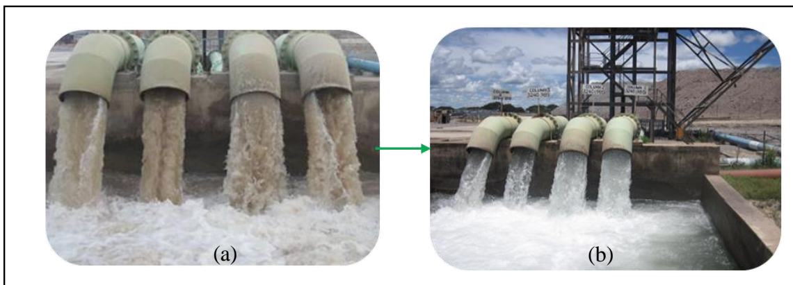
Figure 8.14: Improvement in clarity of waste water as result of reduction in total dissolved solids (Source: Konkola Copper Mines, 2020)
