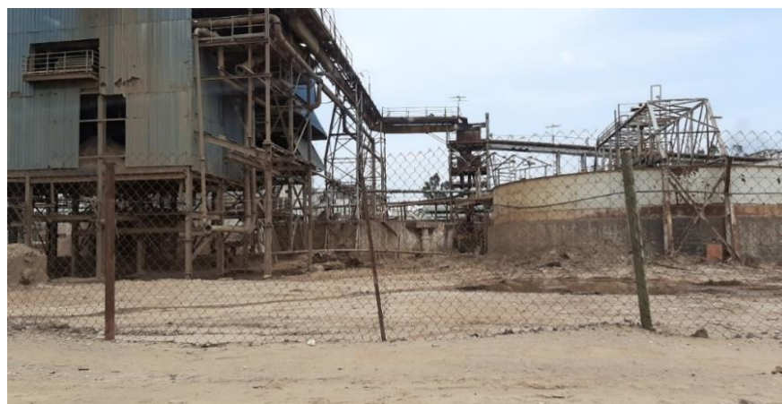
Figure 8.20: Old milling plant at Nchanga mine to be demolished
