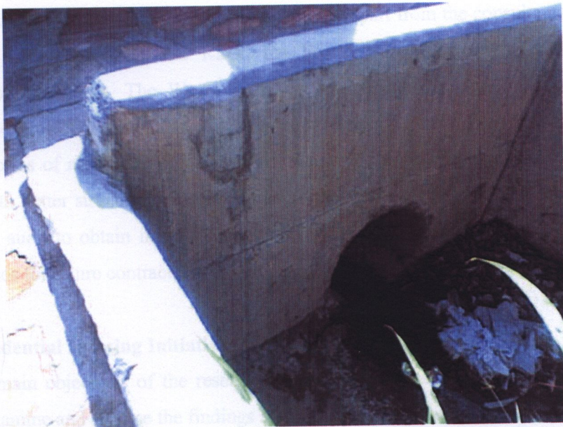
Figure 5.5: Newly constructed headwall along Lusaka – Chirundu Road
