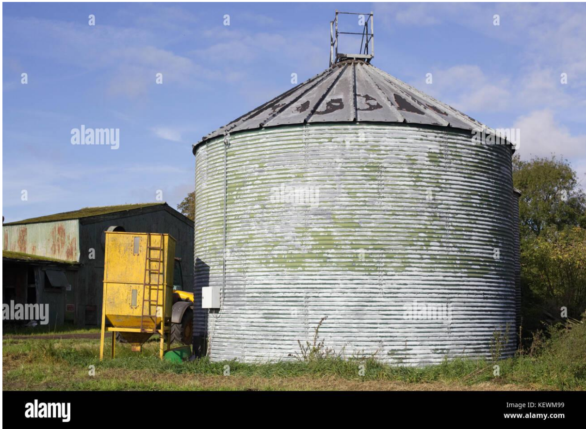
Figure 2.2 A depot in Ethiopia in a dilapidated condition (Source: Internet)
