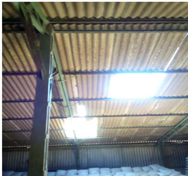
Figure 1.2 Leaking shed
