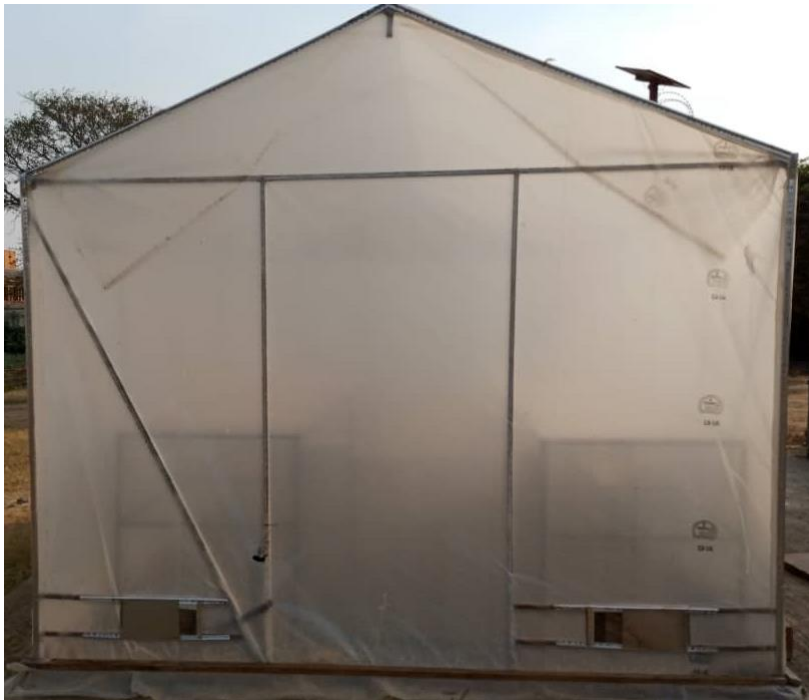
Figure 3. 10 GSD with air vents partially open
