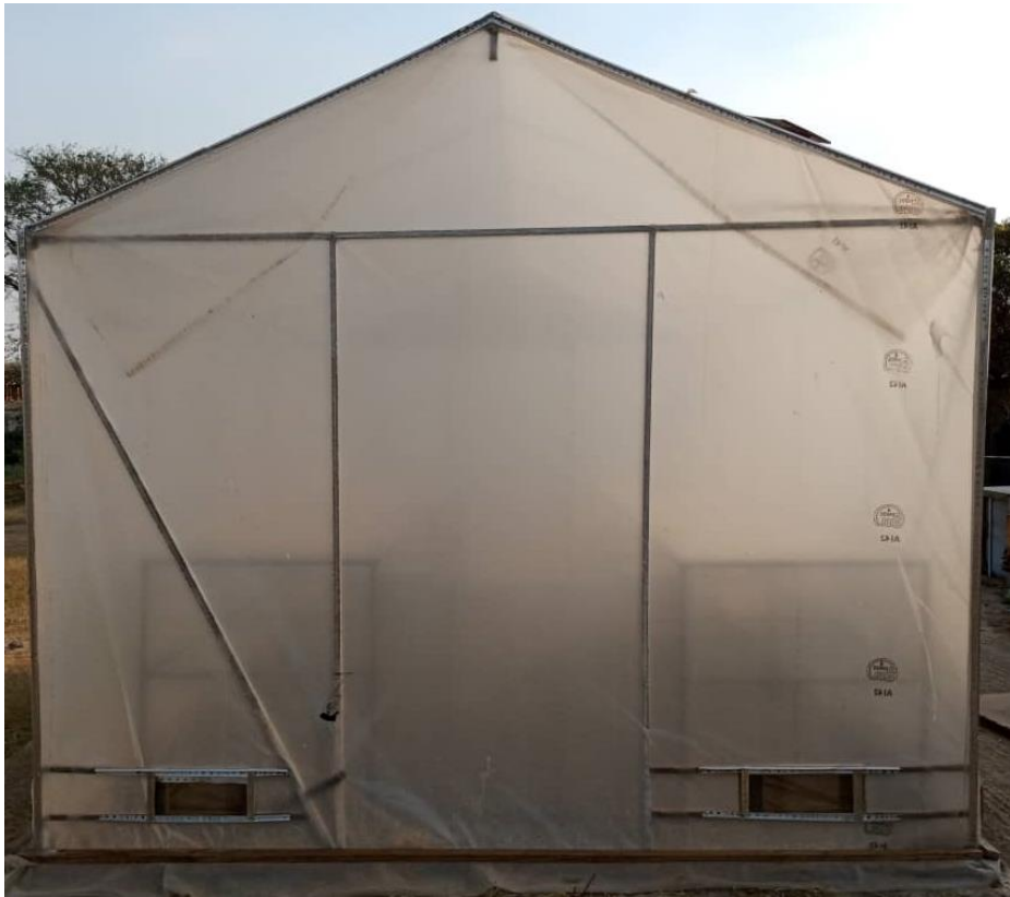
Figure 3. 9 GSD with air vents fully open
