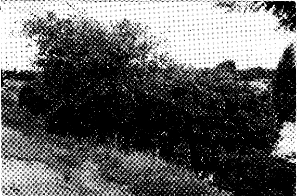
Plate 5.2: Soil Erosion on top of Kalikiliki Dam and trees growing on the Dam
