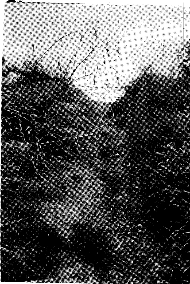
Plate 5.1: Soil Erosion taking place along a human path on the downstream face of Kalikiliki Dam
