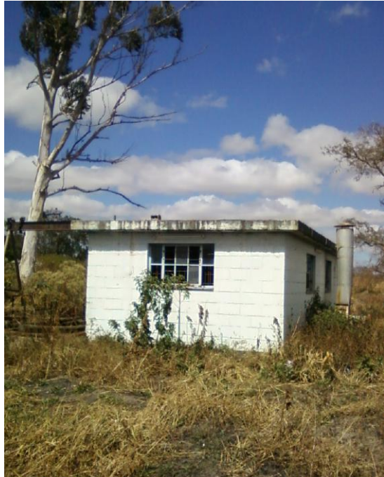
Figure 5.11: UNZA sewerage main pump house near Transport Yard.
