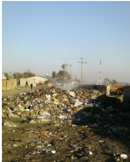
Figure 5.13: UNZA/Kalingalinga wall fence (southeast of campus) on Kalingalinga side.
