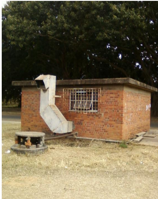
Figure 5.10: UNZA main booster pump house near the Sports Hall.
