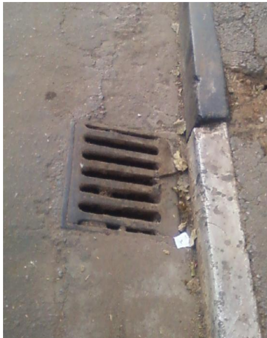
Figure 5.8: A gully (an opening point of a closed drainage system (covered passage)). Source:
