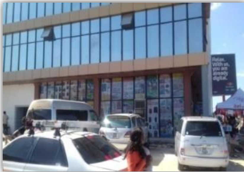
Figure 5.16 A building at a place where land was sold off in Kalingalinga Source: Author, 2017
