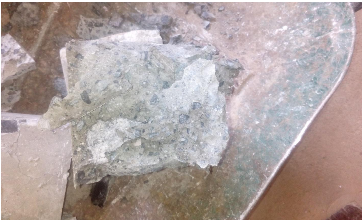
Figure E.6: Failure pattern of heated normal concrete after being subjected to compression forces
