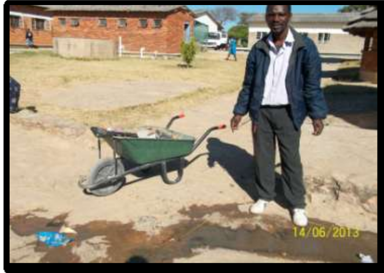
Figure 19: School Sanitary Officer in front of a drain at St. Mulumba Basic School. Source: Field Data, 2013.
