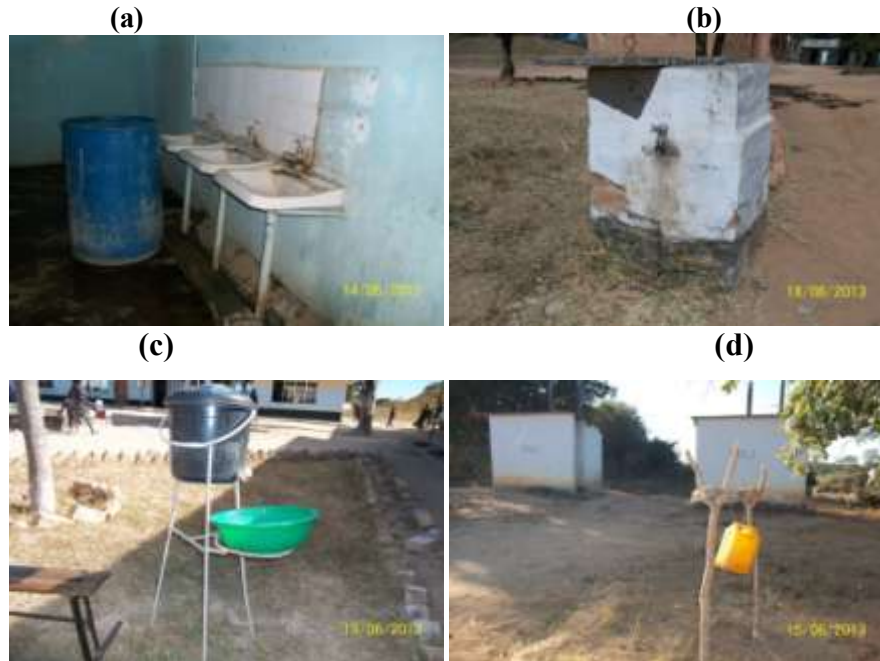
Figure 13: Photographs showing (a) Sinks, (b) concrete tank with tap, (c) Plastic bucket with tap and (d) Plastic container found in Choma Schools. Source: Field Data, 2013.
