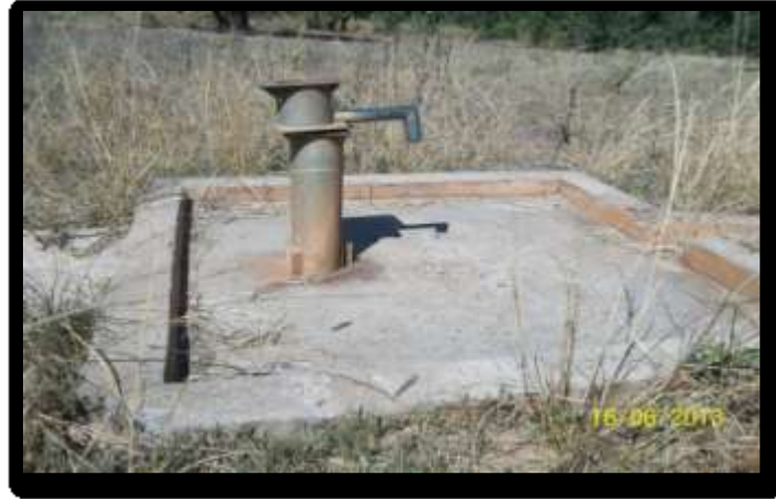
Figure 24: Abandoned hand pump due to lack of water. Source: Field Data, 2013.
