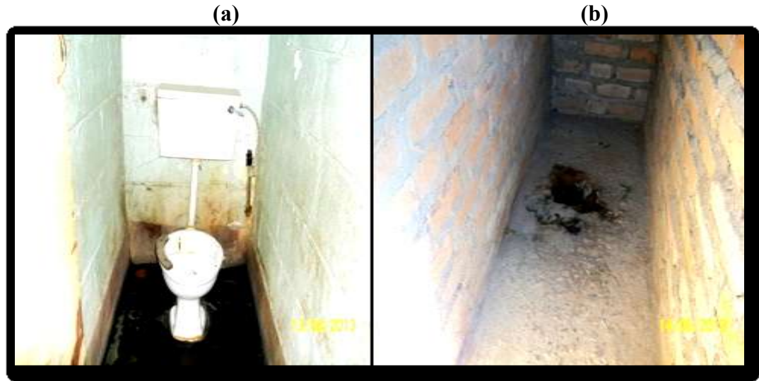
Figure 10: Photographs showing (a) Flush toilet and (b) Pit latrine. Source: Field Data, 2013.
