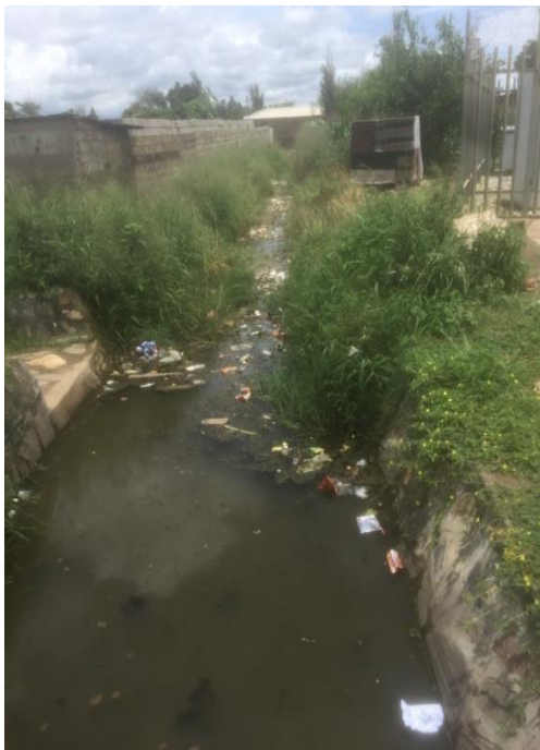
Figure 4. 7: Clogged drainage with waste
