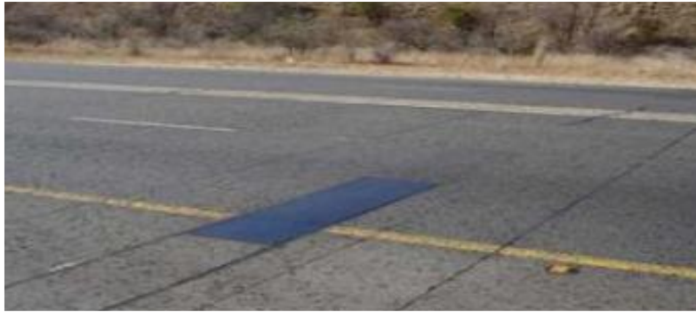
Figure 2.27: Bending Plate WIM [Source: International Society for WIM]
