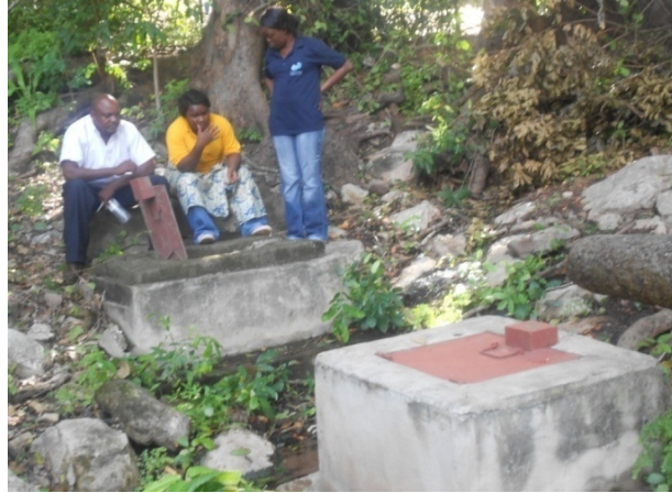
Figure 2: Showing the sealed boxes at the source of Luumbo Spring, Gwembe District, Southern Province, Zambia
