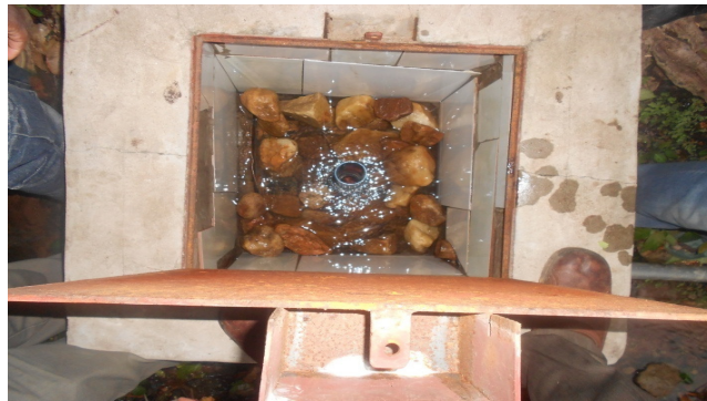
Figure 17: Showing the preliminary treatment point containing stone media in Luumbo area, Gwembe District, Southern Province, Zambia
