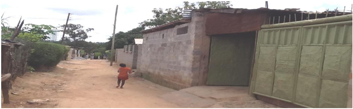
Figure 4.10: Housing transformation through erection of a boundary wall fence
