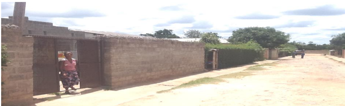
Figure 4.4: Housing Transformation through erection of solid boundary wall fence
