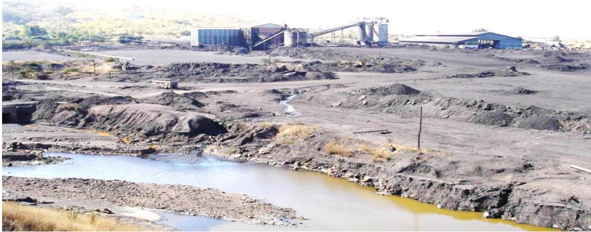
Figure 4.1 The Coal Processing Plant in 2005
