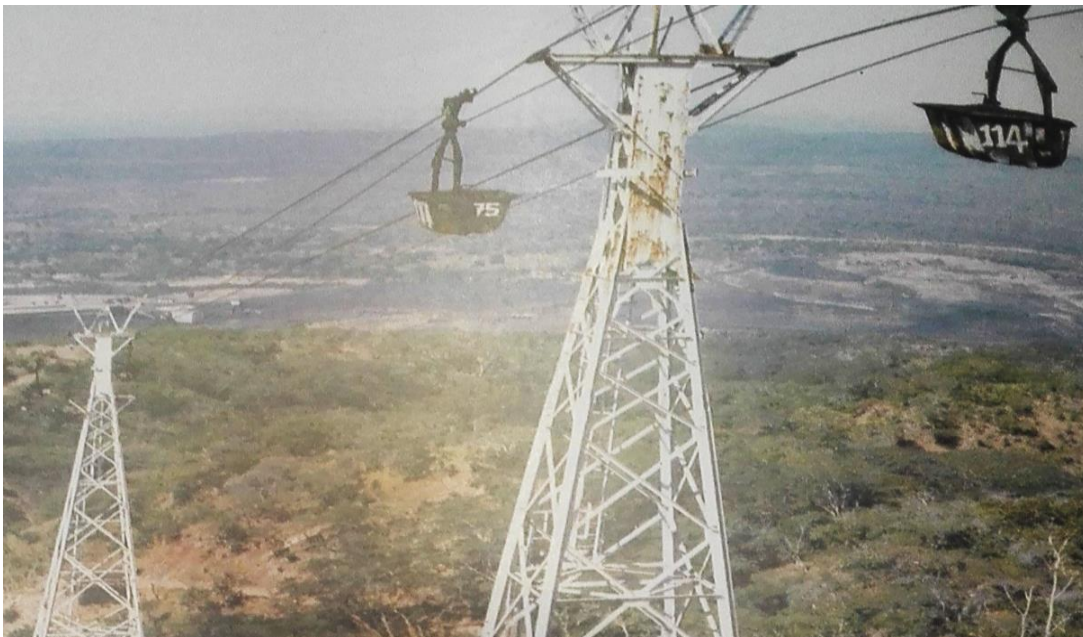
Figure 3.2 Aerial Ropeway at Maamba Colliery, 1988
