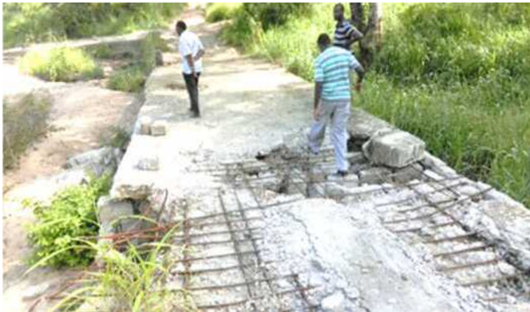
Figure 4.12: Broken Bridge on the road to Chikwa (Chama District). Photo by Doreen
