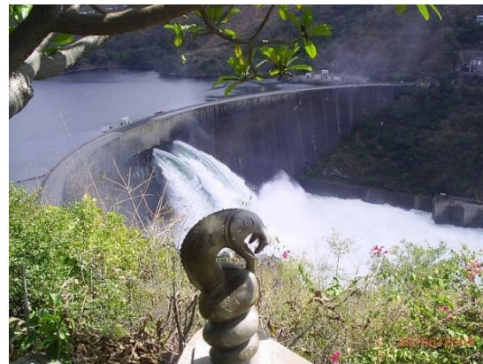
Figure 2. The Kariba dam opening spill gates
