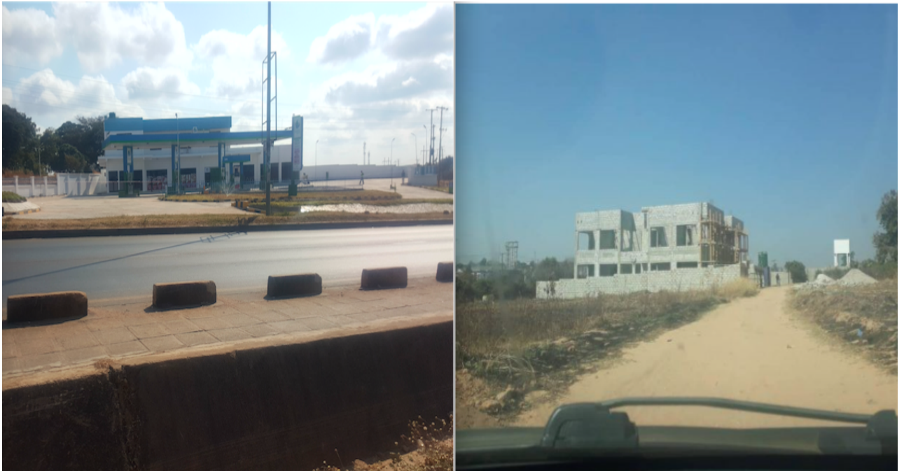
Figure 8. Image shows a filling station and a building at Munali which were spared by the Lusaka province minister.
