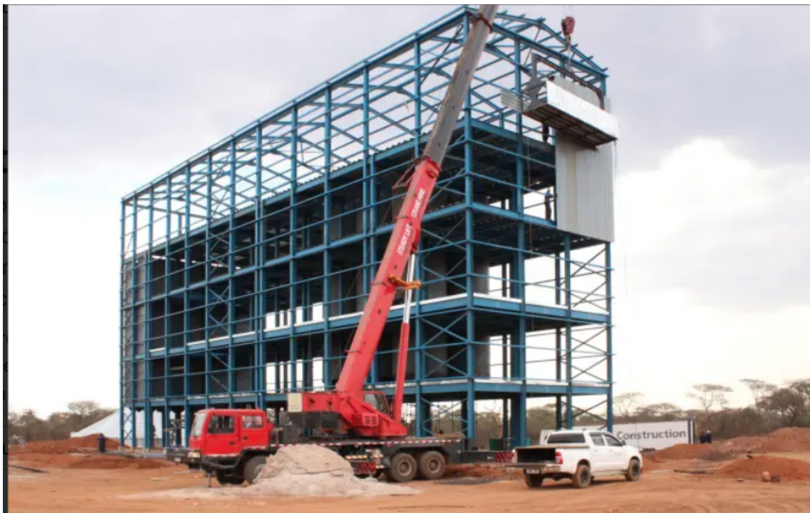
Figure 6. Construction in Chieftainess Chiyaba’s area. (Source field data)
