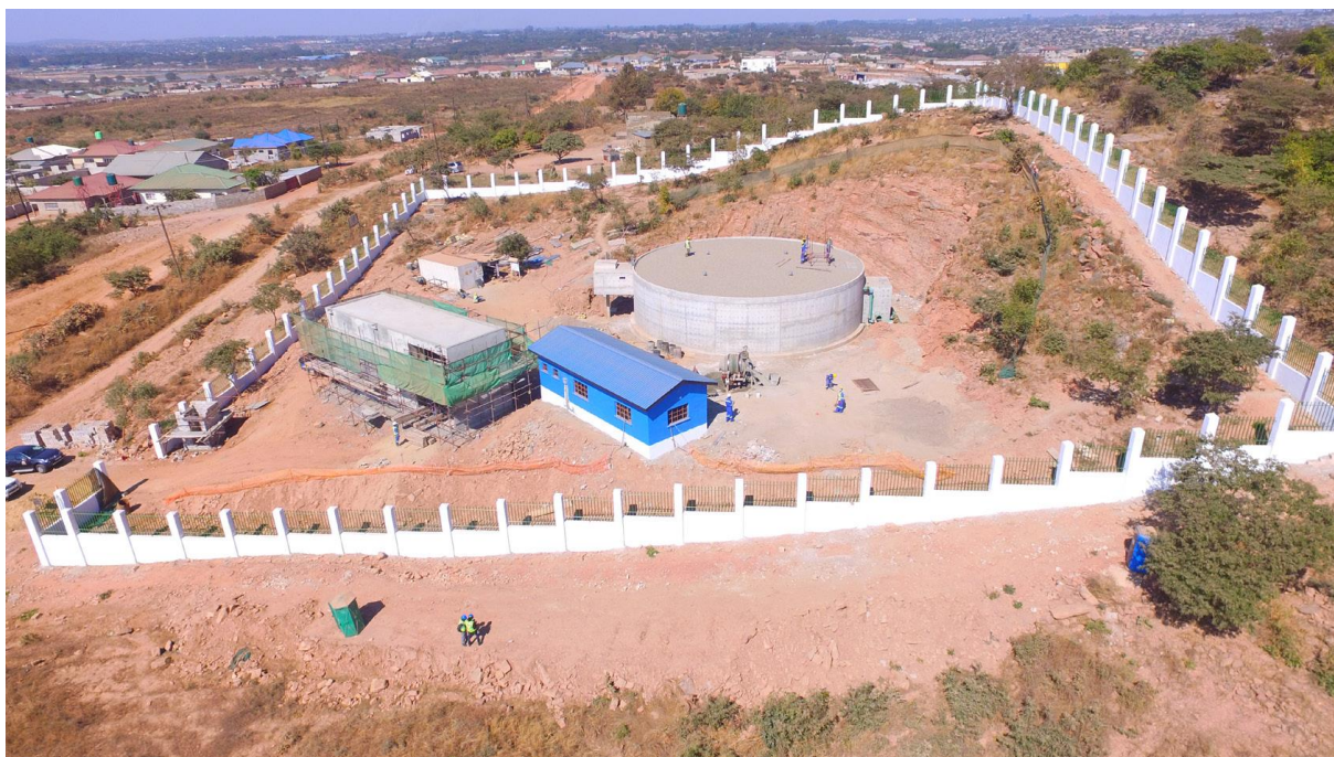
Figure 5.1: Newly constructed water supply infrastructure
